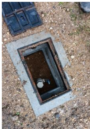
Flush point at the very start of the sewer main at the end of Spencer Rd.
