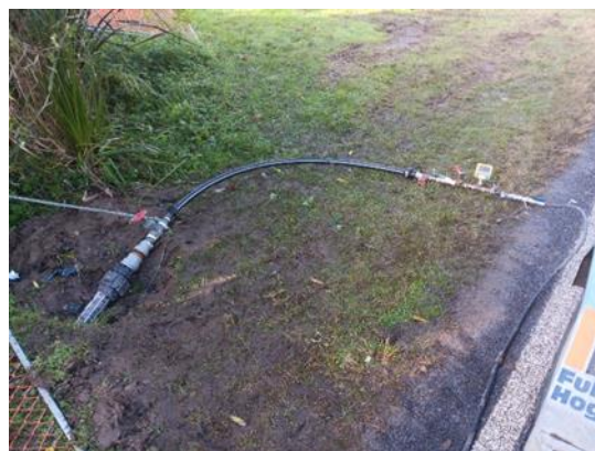
The first 900m section of the main from Spencer Rd to Alexander Rd being pressure tested.
