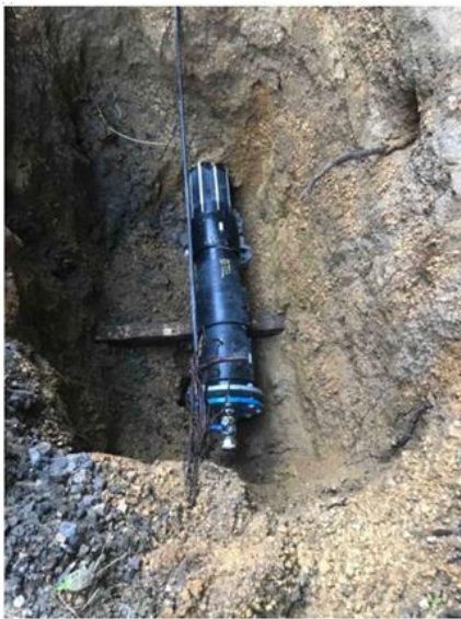
Test End on 225mm Falling Main Pipe, Telecom Cable exposed
