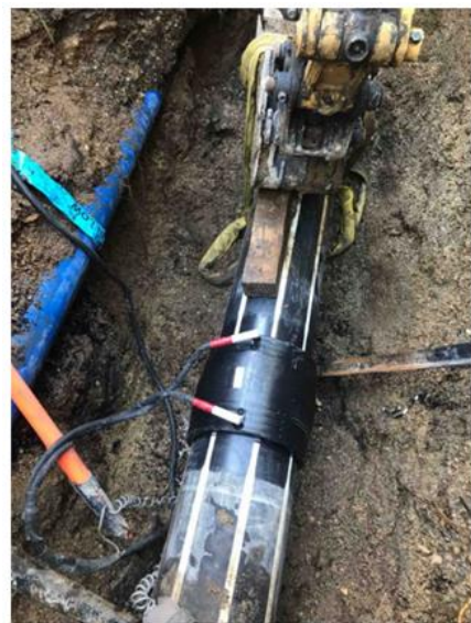
EF Coupler on 225mm Falling Main Pipe
