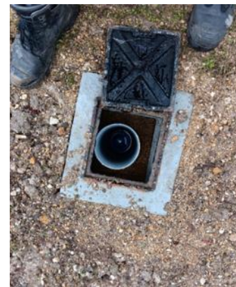
Valve for flush point.
