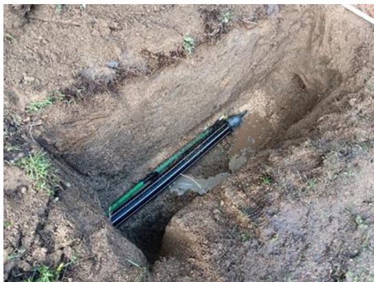
Sewer main alongside electrical conduit for the fibre communication between the pump-stations.
